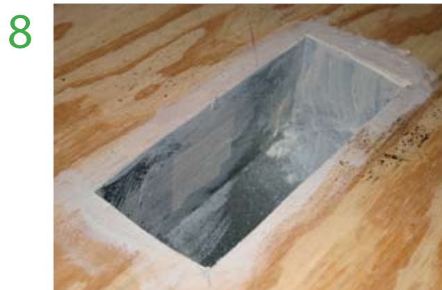
8 Seal boot to subfloor or sheetrock
