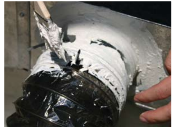
Apply mastic to connection
