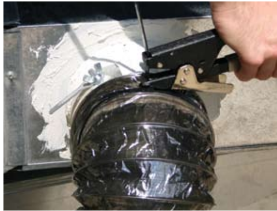
Attach flex duct and zip tie
