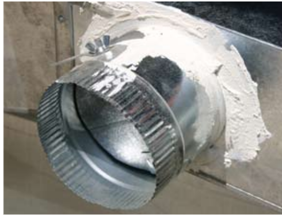
Apply mastic to collar at plenum
