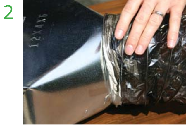
2 Pull liner onto boot
