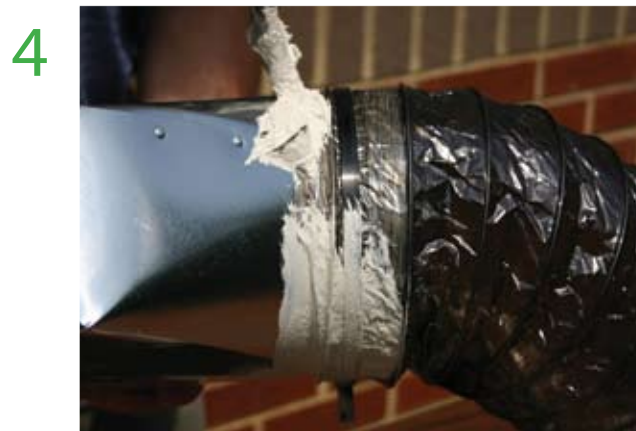
4 Apply mastic to connection
