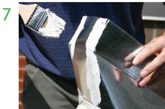
7 Seal exterior seams of boot
