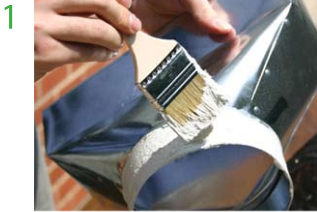
1 Apply mastic to boot
