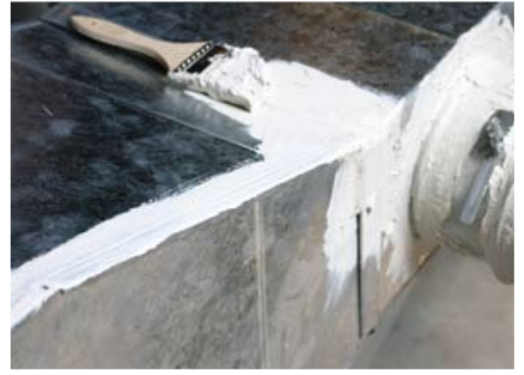
Seal all plenum seams with mastic
