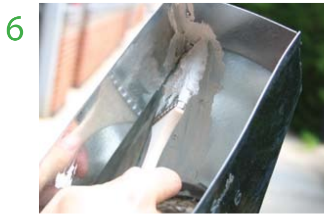
6 Seal interior seams of boot
