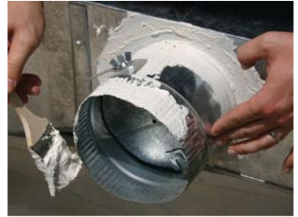
Apply mastic to collar before flex
