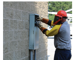
Protective clothing and a face shield are some of the many ways an arc flash injury can be prevented.
